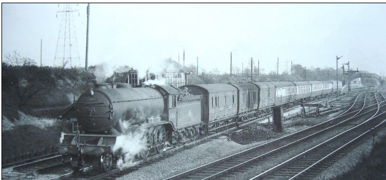
1956 Annesley North junction box behind the train and Hollinwell & Annesley station and bridge in distance.
