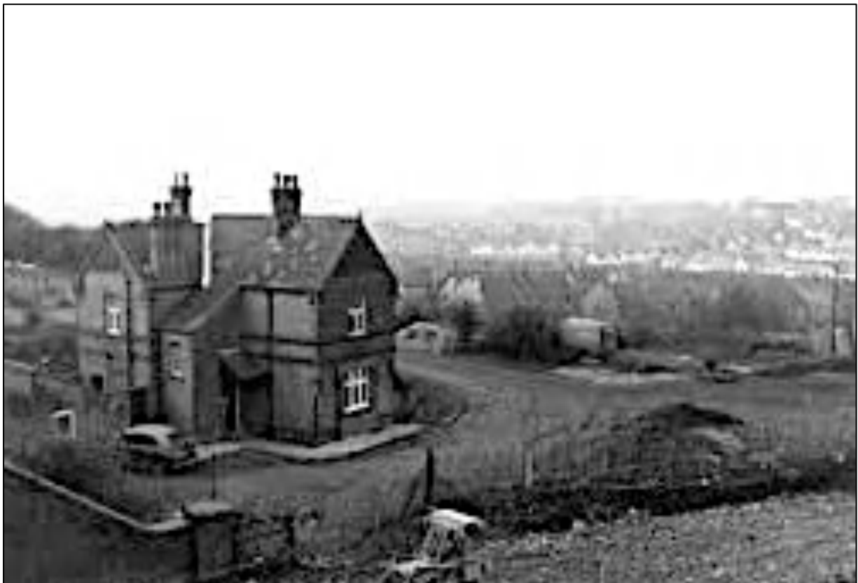
The Bulwell Common Station after it closed. It is now surrounded by houses.
