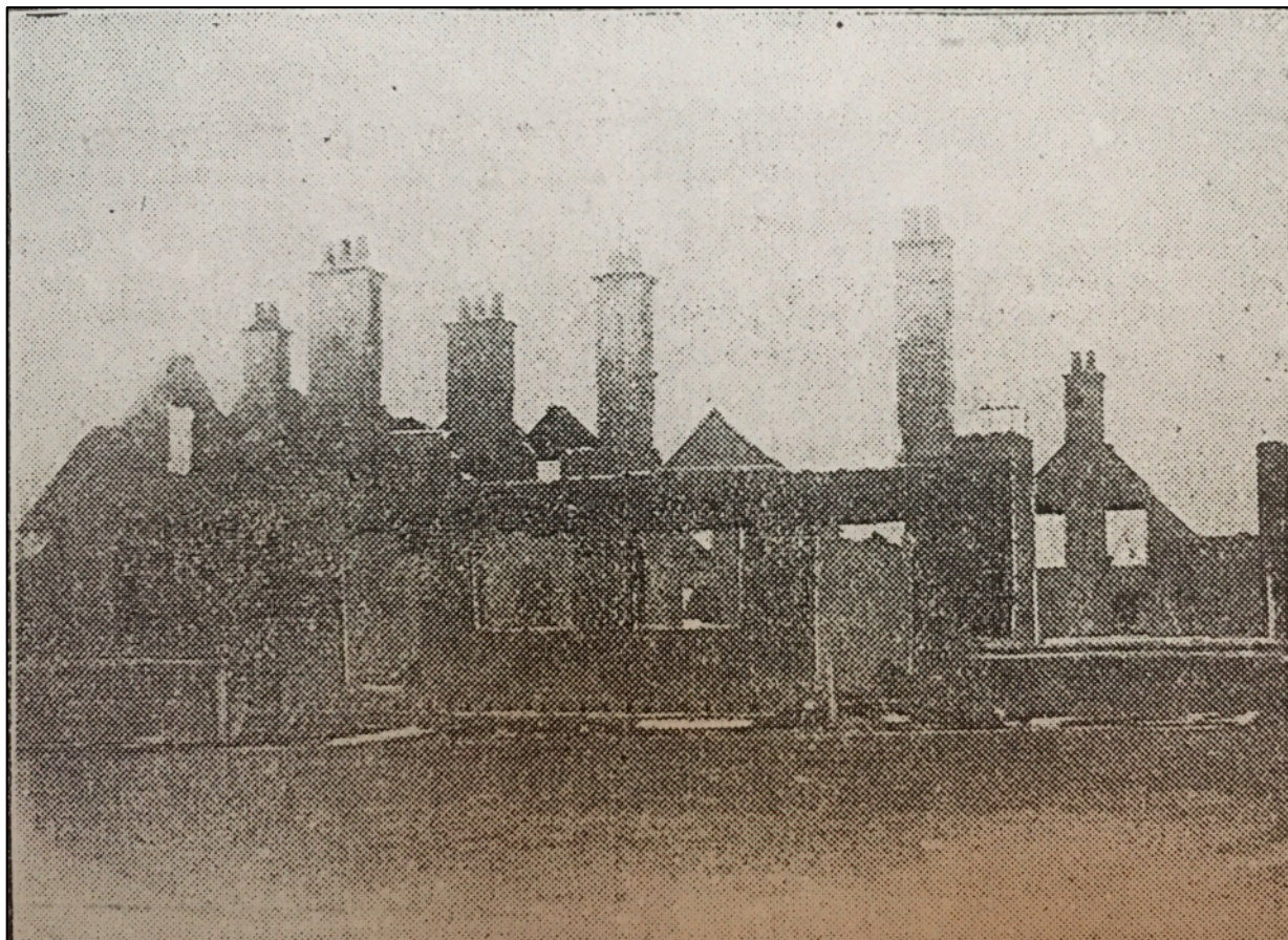
11.1.1924 Burnt out clubhouse.
