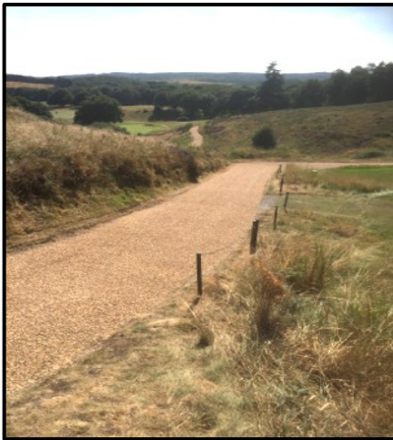
2016 Epoxy resin path 13 th hole.
