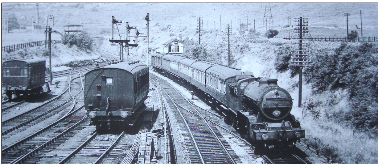
1958 Annesley tunnel just visible with Annesley North junction box on right, Robin Hood Hills in the background.
